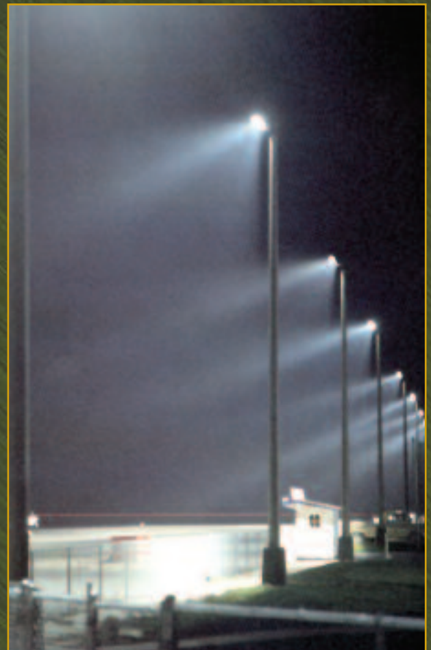
Demonstrates house side spill light control.
